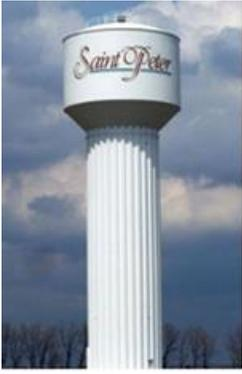
**BROADWAY WATER TOWER WORK** - The 1984 Broadway Water Tower, which has a 500,000 gallon storage capacity, is scheduled for structural repairs, sand blasting, and new painting of the tower and logo early this summer. City staff inspects the tower each year looking for defects and to ensure the
